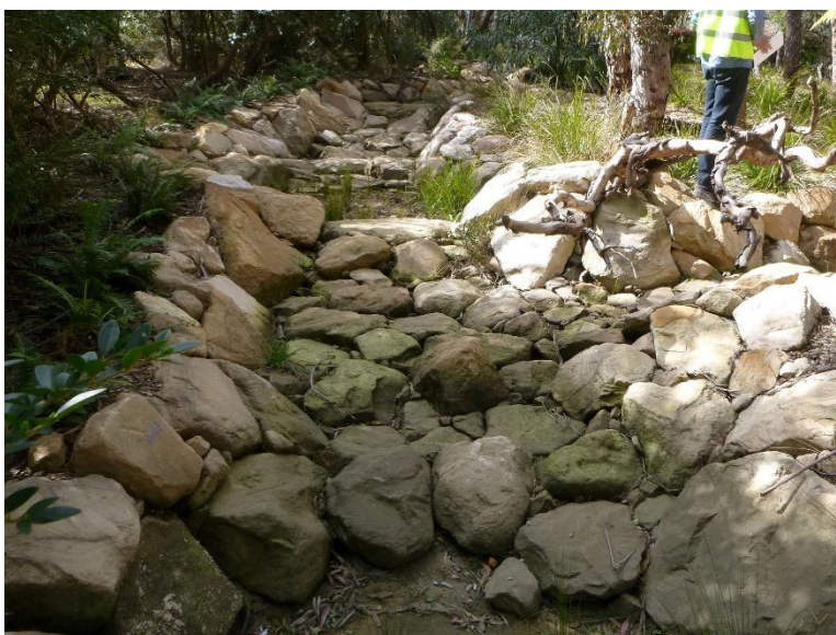
Canberra St Wentworth Falls Stormwater Biofilter (Paul Vale)
