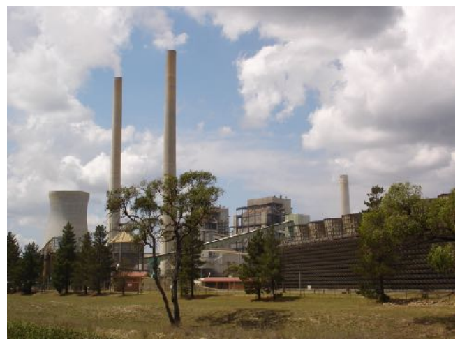
Wallerawang power station. In 2007 it was producing coal-fired power but in 2021 it has been mainly a prop for a reality TV program. In the post lockdown period, are infrastructure decisions going to be forward looking or backward looking? (Source: Andy Mitchell (Amitch) - Own work CC BY-SA2.5, 2007)
