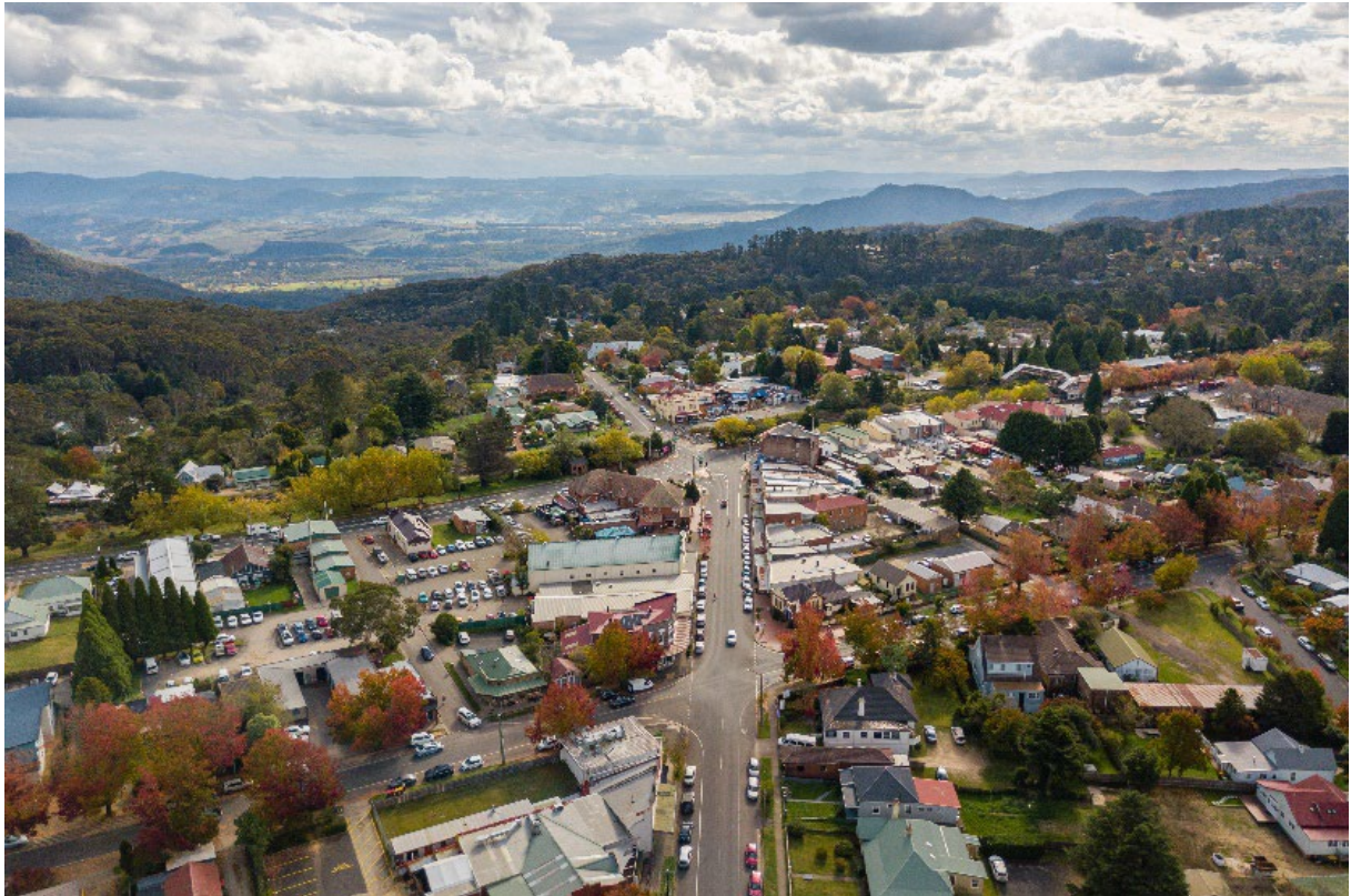
Aerial image of Blackheath
